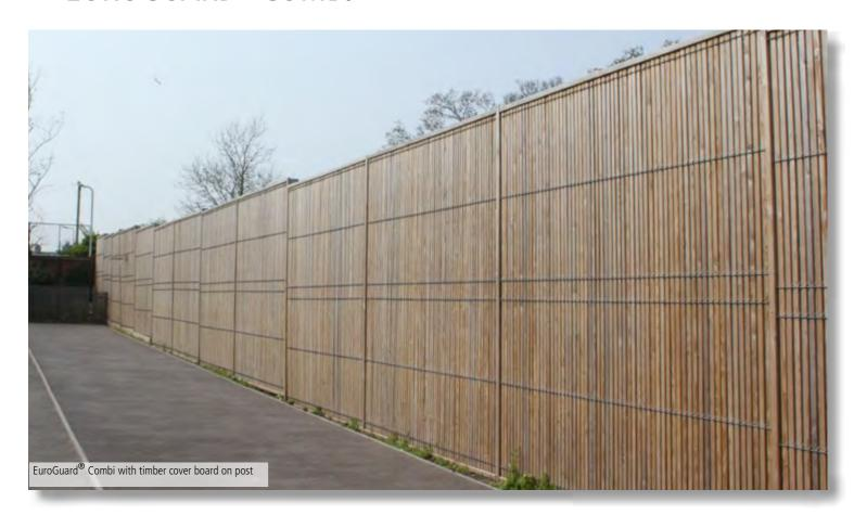
EuroGuard® Combi brings our experience and reputation in steel and timber fencing and gates together in a design that combines the beauty of natural wood with the strength of steel. The robust fence panels and matching gates provide the additional advantages of a flat facing surface with no hand or foot holds as well as closely spaced slats for added privacy.
