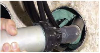
4. Further fill around the services, pushing hard to ensure full compaction and to within 50 mm of the wall
