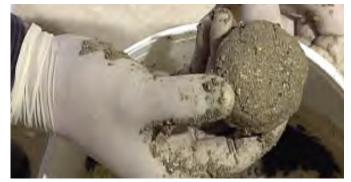
6. When fully mixed, form a ball or mortar. Add more water as required until the ball is stable and does not fall apart
