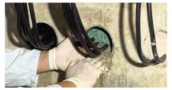
7. Push the mortar tightly into the sleeve to the wall surface to fill the remaining 50 mm of depth with mortar
