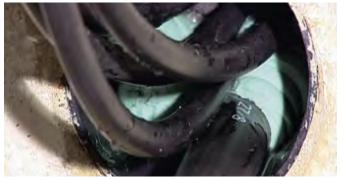
3. Slightly elevating the services, inject about 100 mm of sealant, slowly pulling back ensuring that all voids are filled
