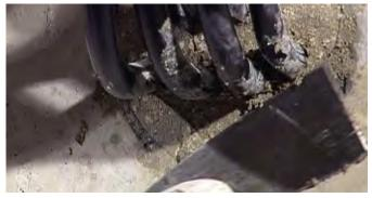
8. Smooth the face of the mortar with a small scraper, adding a little water to assist
