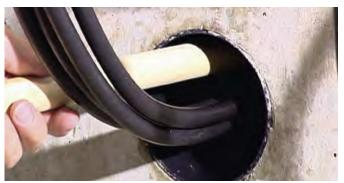
2. Insert a piece of foam to act as a back-stop, pushing into the duct with a stick so that it is 150 mm in from the wall surface
