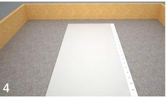
The membrane is fitted to within 50mm of the top of the vertical raft temporary formwork. Mark out the height of the fold onto the membrane, marking out twice the height of the upstand, creating a guide for the fold.
