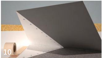
Seal the 45 degree joint with the double sided HydroBond tape. Use a hard roller to ensure a firm bond of the tape to the between the two surfaces of membrane.
