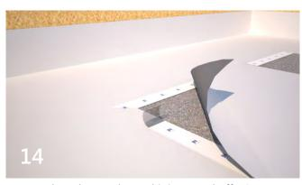
To complete the overlapped joints, peel off BOTH OF the protective release linerS from THE FRONT AND REAR SIDES ALONG the adhesive edge of the HydroBond Tape and press the laps together. Use a hard roller to ensure the laps are fully and constantly adhered.
