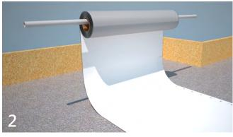
Unroll the membrane with the geotextile towards the concrete to be waterproofed (white fleece facing up) using a long scaffold pole or similar.
