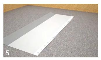
Fold along the guide created in the previous stage. Sharpen the crease with a hard roller.
