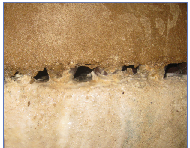
Figure 4: When limescale completely blocks a Type C system, leading to complete system failure
