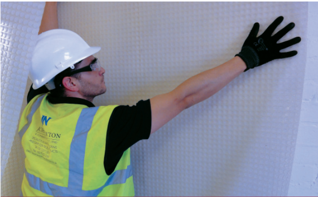
2 Place the membrane to the wall
