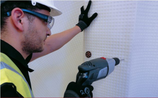
4 Drill and then fix with the fixing plug
