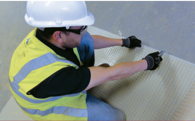
1 Cut the membrane to size
