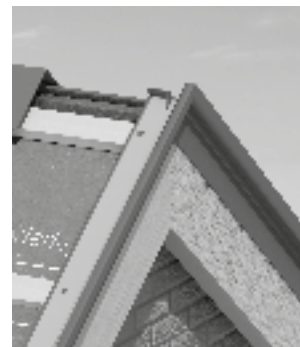
Fig. 27 – Interlock left and right hand trims
