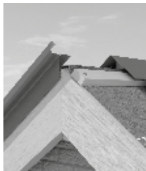
Fig. 26 – Nail left hand trim in place
