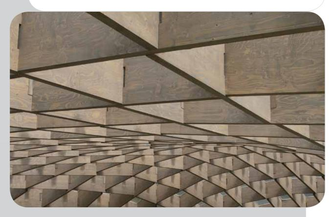
Cetol HLS plus has been extensively used on the interlocking timber beams of the visionary Serpentine Gallery Pavilion in Kensington Gardens, London, to provide the flexibility of protection needed in areas of particularly high movement.
