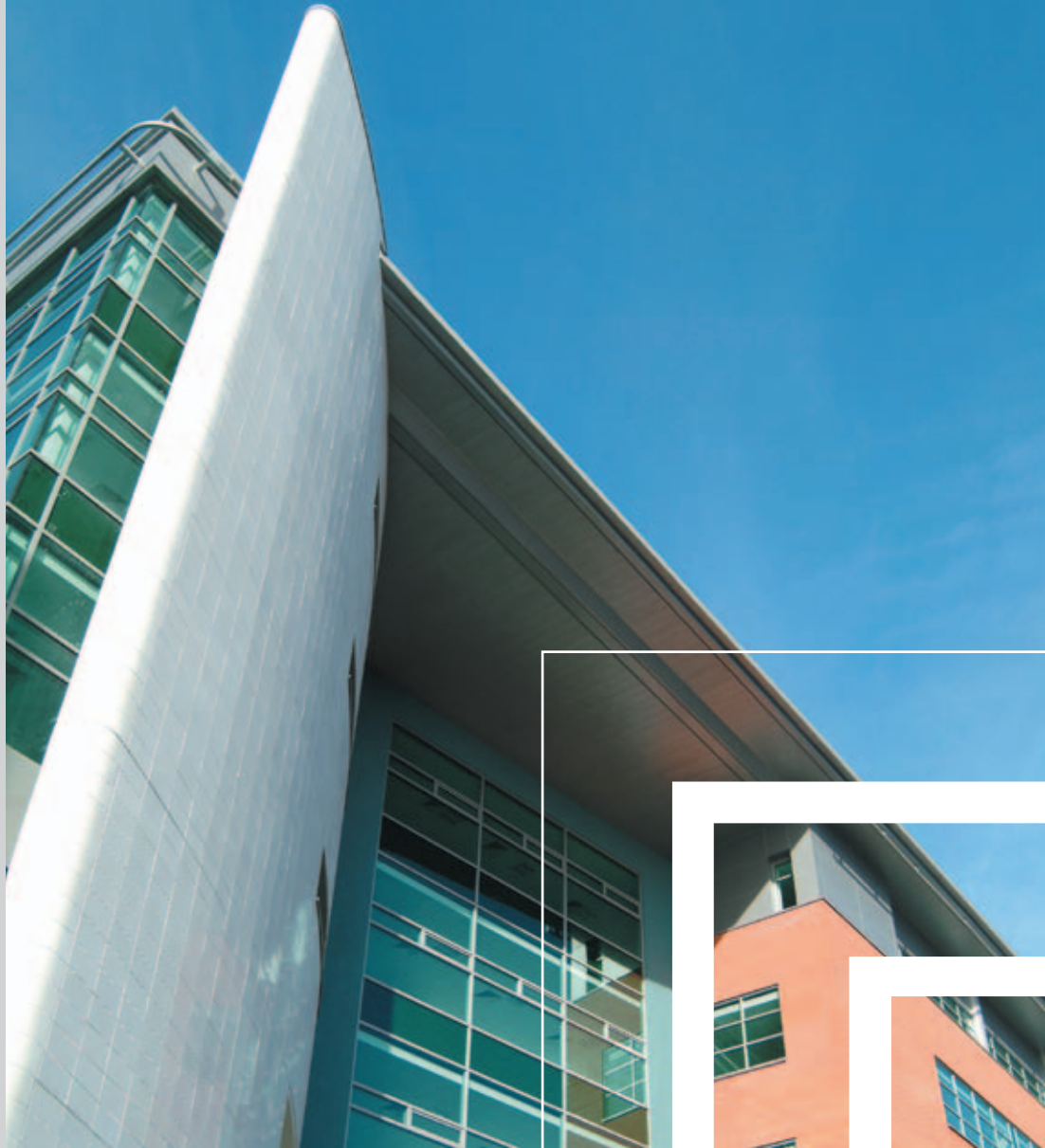
Medici masonry, Twelve Princess Dock, Liverpool
