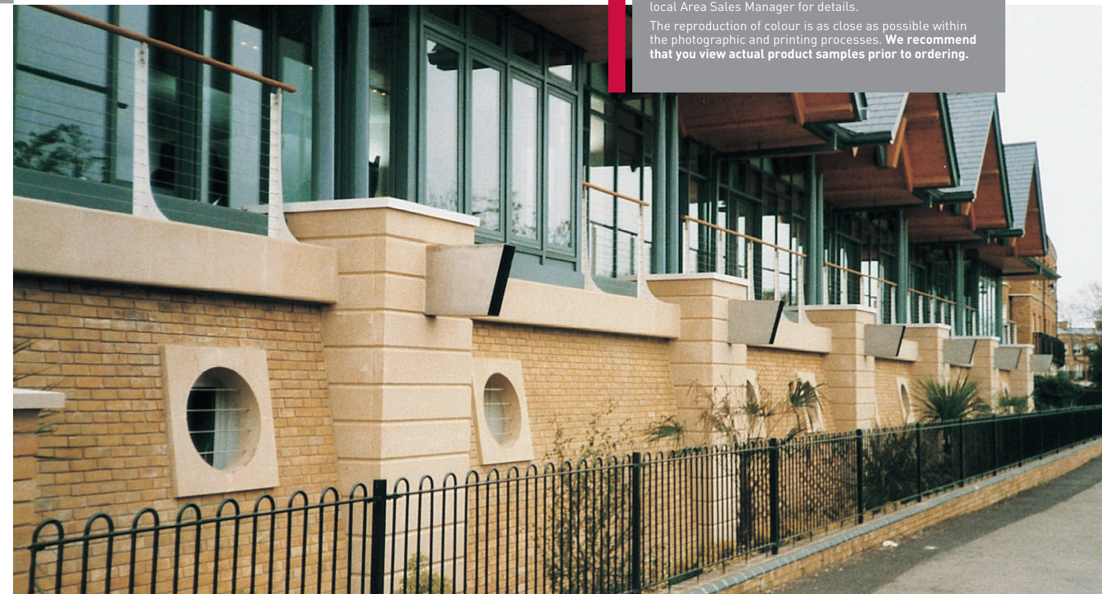
Cast Stone at Weir House, Tameside.
