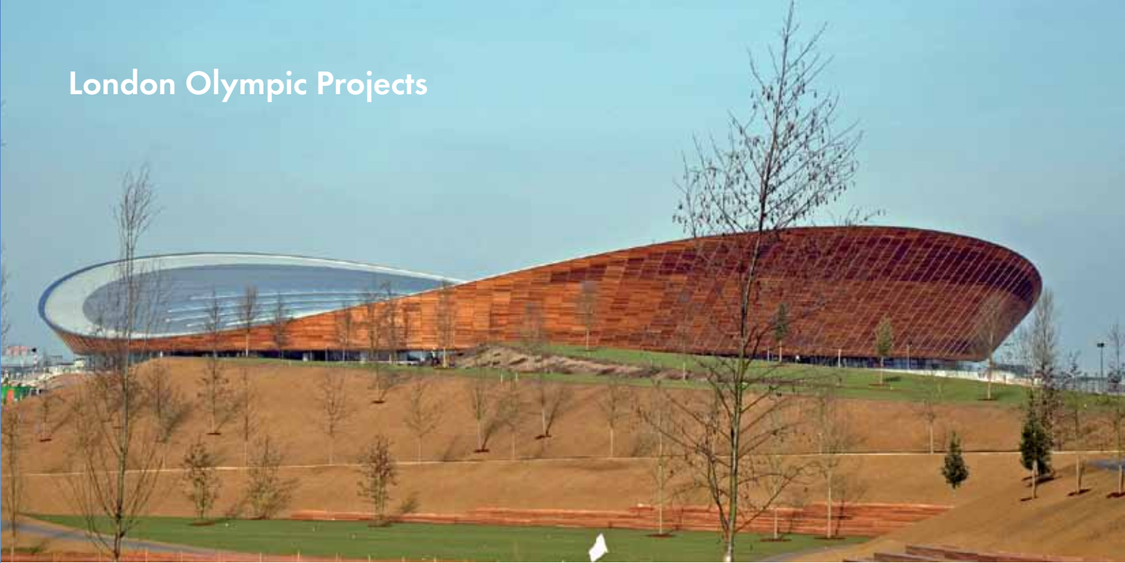
The Velodrome, Architect: Hopkins Architects
