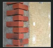
BrickShield® Special-shaped Clay Brick Slips are available for corners and reveals.
