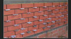
BrickShield® Adhesive Mortar is then applied to the surface of the Rockwool® Façade Ultra. BrickShield® Natural Clay Brick Slips are laid onto the adhesive mortar, keeping to line and level for an even appearance.
