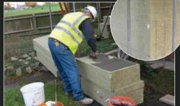
Rockwool® Façade Ultra coated with BrickShield® Adhesive Mortar is then applied to sound, dry and smooth masonry.
