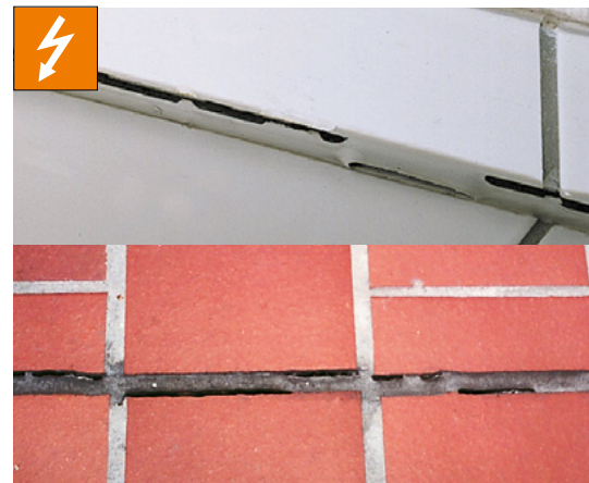
This type of damage is preventable with Schlüter®-DILEX movement profiles.
