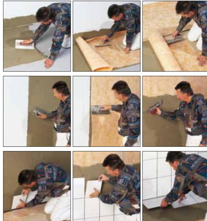
1. The area to be waterproofed must be clean, even and load bearing. Cut Schlüter®-KERDI to the appropriate size using scissors or a utility knife.
