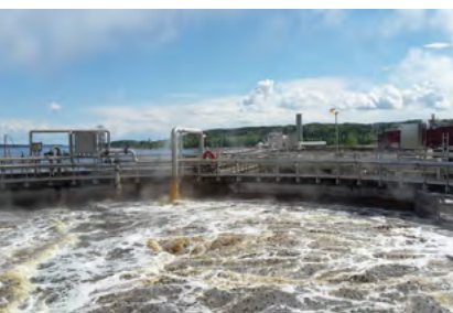
Fig. 9 Wastewater treatment in a pulp mill.
