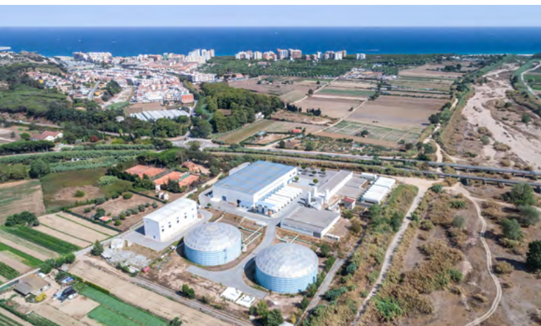
Fig. 11 Desalination plant at the seaside in Spain.
