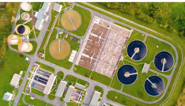
Fig. 6 Wastewater treatment plant.
