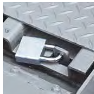
Recessed padlock hasp covered by a flush hinged lid
