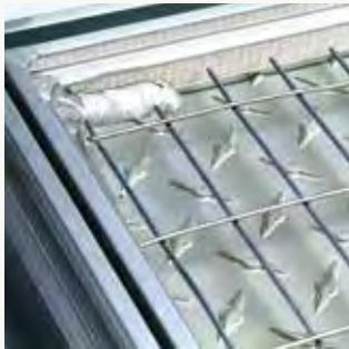
Top side - ready to accept floor finish
