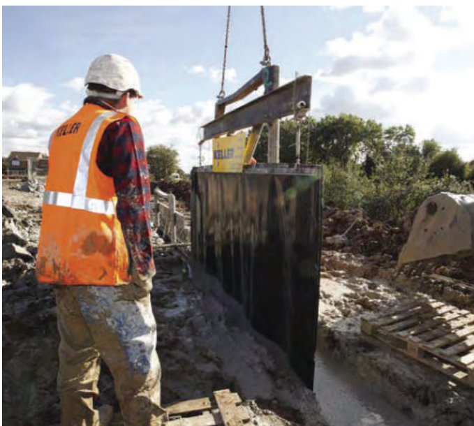
Gravel trench being constructed using temporary support provided by bio polymer muds.
