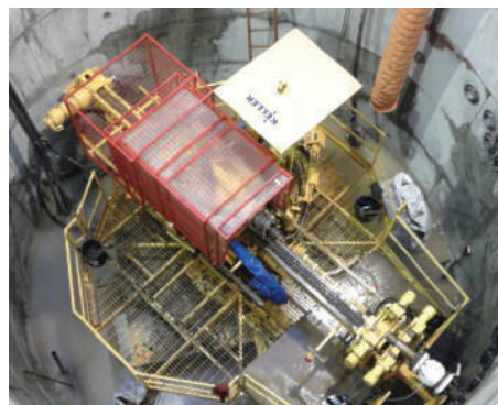
Drilling within a shaft for installation of Compensation Grouting pipes.
