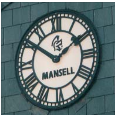
A Skeleton clock with company name and logo added to the dial and internally counterbalanced hands.
