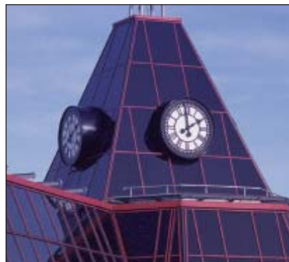
Special 2400mm clock enclosures with 1800mm Skeleton dial back illuminated clocks.
