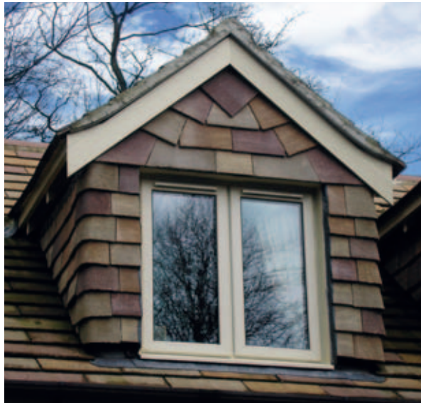
Hardrow® Slates Harmonies® in Concerto, Orion Homes. Vertical tile cladding and external angles.
