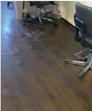
Damage due to residual moisture.
