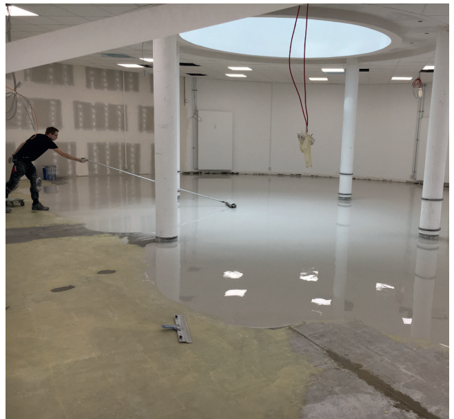
High strength class CA-C35-F7, fire class A1 fl , hardly any usage restrictions – UZIN NC 110 NEW can be employed wherever unstable substrates require a low-tension smoothing compound.
