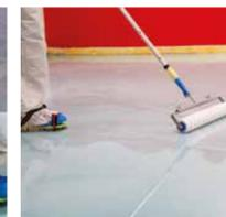
In the last step the second sealing coat is applied
