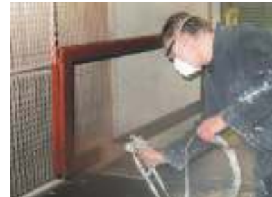
Anti-rot and anti-fungal treated with a low maintenance spray finish.
