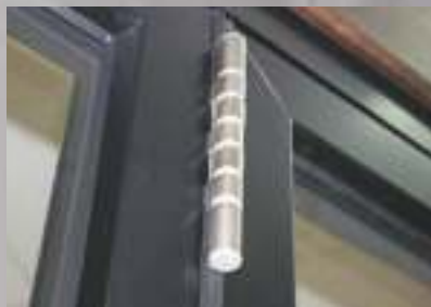
High security hinges, non face fixed.
