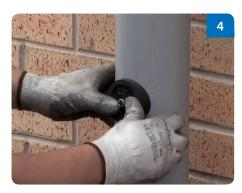
Insert the Access Point into the hole so that the curvature of the seal follows the curvature of the main pipe.
