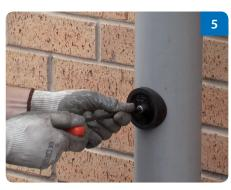
Fix the Access point to the pipe using the 6mm Allen key supplied.
