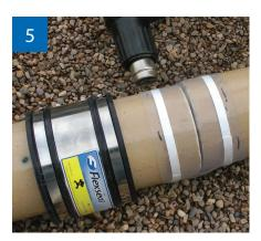
Slide the FEP liner over the seals and apply hot air evenly to shrink it onto the pipe
