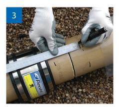
Mark off the positions for the PTFE seals symmetrically, to ensure they are directly underneath the clamp bands
