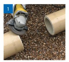
Ensure the pipe ends are free from debris and chamfered to a minimum of 3mm x 45°
