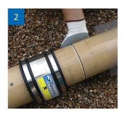
Slide the sleeve and coupling onto the pipes and butt the pipes together
