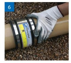
Position the coupling centrally over the liner and tighten to the recommended torque
