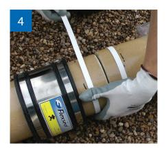
Fit the self adhesive seals onto the pipes, overlapping the tape ends
