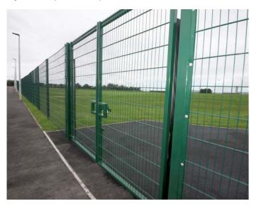
A feature gate manufactured to designs developed from a concept provided by the school and architect, and one of the swing gates installed within the 2.5 miles of fencing
