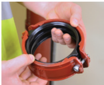
1. Slacken bolts on coupling to fullest extent to ease assembly.
