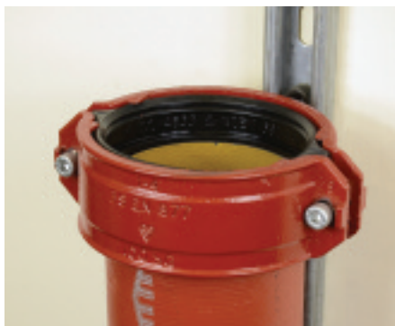
2 Push coupling over the end of the pipe or fitting ensuring the central register is abutted against the spigot edge.
