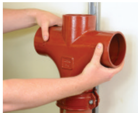
3 Push the second pipe or fitting into the coupling again ensuring that the spigot is abutted against the central register.
