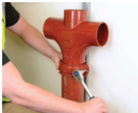
4. Check alignment of assembly before tightening the bolts. Coupling bolts on all sizes are M8 and require special Allen socket adaptor (6mm) EF102, together with a ratchet spanner EF100. Alternatively use a time saving power tool.
