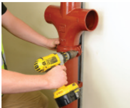
4. Check alignment of assembly before tightening the bolts. Coupling bolts on all sizes are M8 and require special Allen socket adaptor (6mm) EF102, together with a ratchet spanner EF100. Alternatively use a time saving power tool.
