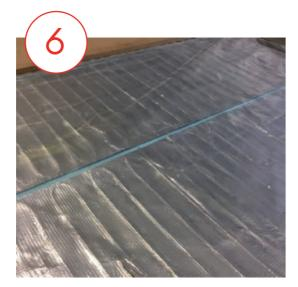
6. The floor finish can now be installed. Always install the floor finish in accordance with the manufacturers requirements. Ensure the flooring is suitable for use with underfloor heating and has been acclimatised to the room following manufacturers guidelines before installing. Leave room for expansion around the edge of the room if the flooring manufacturer states this is required.
