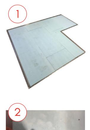
**1.** Before installation, the subfloor must be clean, dry, level and all protrusions removed. Lay the Gaia-XPS insulation, ensuring the whole floor is covered. To prevent movement, fasten with tape, DO NOT use any type of spray adhesive to stick the insulation down.
