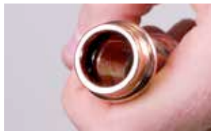
6. Ensure the O-ring is seated
