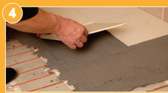
Cover with a layer of self-leveling compound/flexible tile adhesive and allow to dry before tiling. Alternatively lay the adhesive and tiles in one step ensuring the cable is totally encapsulated to prevent air gaps.
