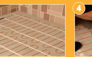
When satisfied with the proposed layout fix the matting to the floor using the integral self-adhesive fixing strips.
