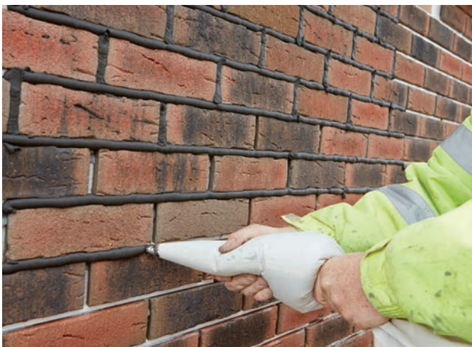
Applying mortar
