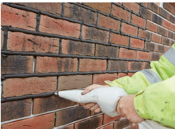
Applying mortar
