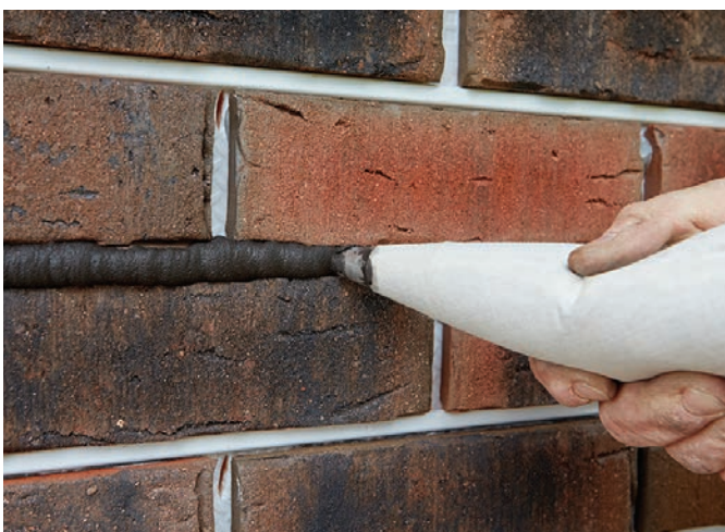
Applying mortar
