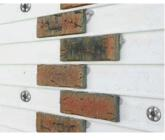
1. The ribbed backing panel is fixed to the substrate. (Fixings vary according to substrate.)
