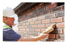
**6.** Once the mortar has set but not dried the brickwork is brushed to finish.
