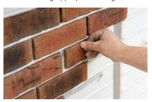
**3.** Brick slips are pushed into place leaving 8-12mm perpendicular gaps between bricks.
