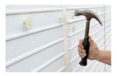
1. System backer panel arrives as one composite sheet. The panel is fixed to the substrate using appropriate fixings.
