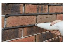
**4.** Specially formulated mortar is then piped into the brick joints.
