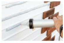
**2.** Permanent bonding adhesive is gunned in continuously towards top of course.
