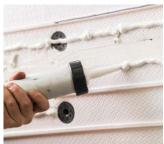
6. Apply a generous bead of high grab adhesive ¾ of the way up each standard course, ensuring the fastener head is covered. For a double or triple course sized slip, use 2 or 3 beads of adhesive respectively.
