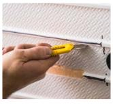
4. Carefully cut away the ribs to create a flat surface for the larger stone slips.
