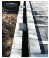
Telescopic adjustable ventilators (Type TAV) (to ventilate underfloor areas) have been built into the exterior cavity wall prior to bedding of the perimeter Cavicloak. Each ventilator has been extended in height to take advantage of the Cavicloak bedding level coinciding above it and providing protection. This approach removes the necessity to individually protect each ventilator at a lower course level.
