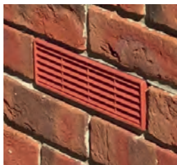
Radon evacuation from structure via Cavibrick located under Radon cavity barrier level.
