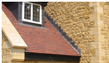
Multicourse Regular Wide Front to Back Dimensions. The natural hamstone is built against a concrete backing block resulting in an external leaf of 250mm thickness beyond which is the cavity. Thus the trays have extended front to back dimensions.
