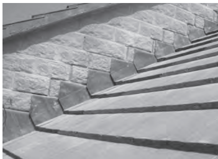
Multi-course Cavitytrays installed in 150mm (6inch) steps. In this example trays have been inserted into an existing wall, demonstrating masonry removal is minimal.
