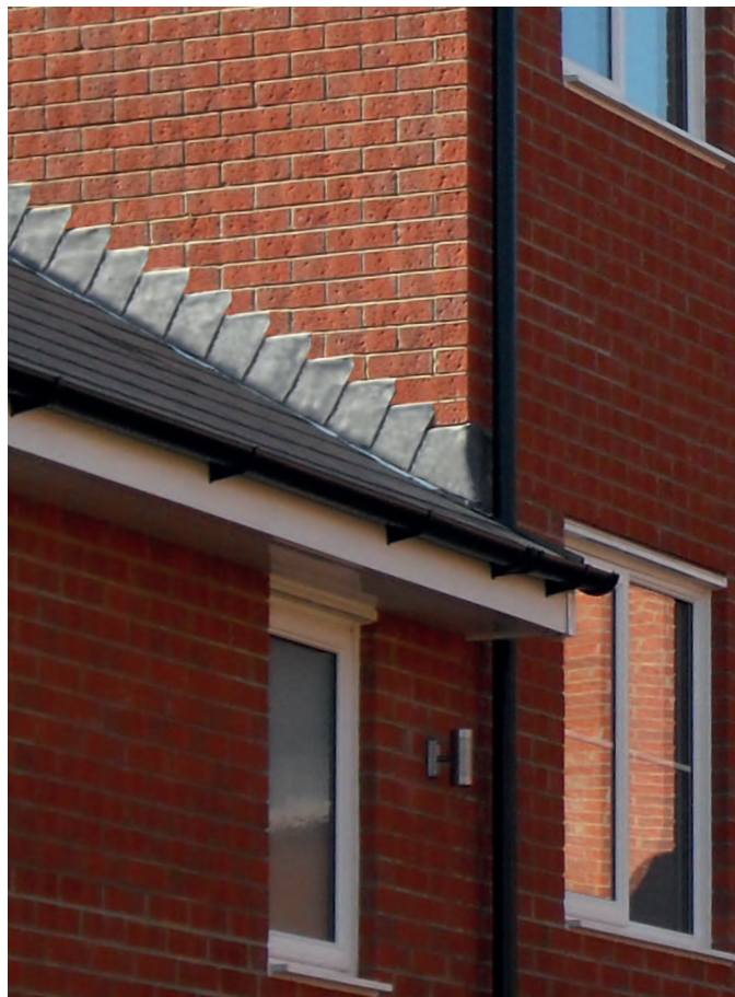
Type CRSS Continuous Running Soaker Strip at slate/wall junction with Type X Cavitytray flashings dressing over CRSS upstand
