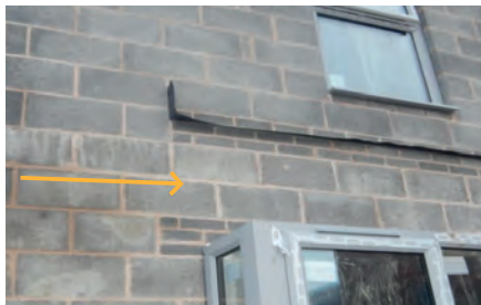
The greater the distance between lintel level and roof intersection DPC/tray level, the greater the susceptibility to damp permeating horizontally across the bay.
