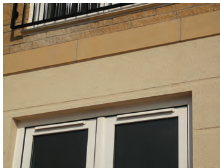
When closing reveals the opportunity exists to maximise thermal retention and consistent protection as the dpc is preformed and not susceptible to distortion or misplacement.
