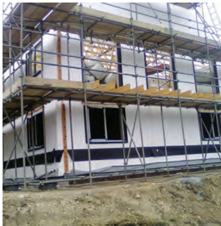
Bespoke preformed insulated DPC surrounds for openings supplied for use on German system building developments
