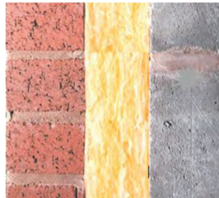
Leaving the insulation projecting the reveal and cutting it vertically afterwards is an alternative approach.
