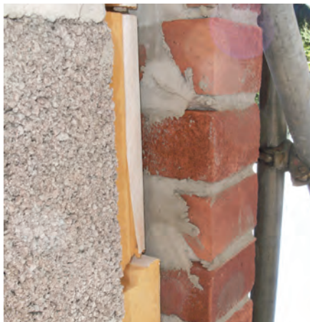
Full fill modular insulation is commonly out of alignment or finished too far back from the reveal face. Consequently there are gaps (hidden from view) between the insulation and a conventional cavity closer
