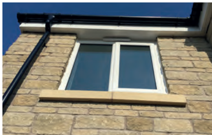
Protection of jointed sill (NHBC 6.1-S4d)
