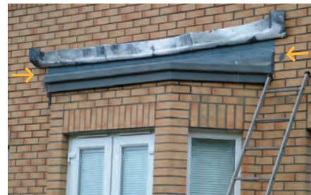
The extensive fascia height means there are a considerable number of masonry courses between the bay support lintel and the higher roof/tray intersection level. To prevent damp permeating between the two it is necessary to incorporate a vertical link whilst maintaining coursing and bond.
