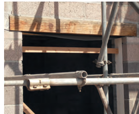
Opening ready to receive 2nd fix Quickcloser
