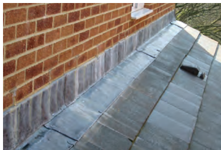
Flexible cavity upstand can accommodate the as-built cavity width
