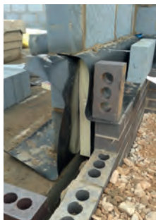
The design detail and the resultant as-built detail, demonstrating the necessity to rely on support from a convenient inner skin course can result in the arrangement being rather cumbersome.
