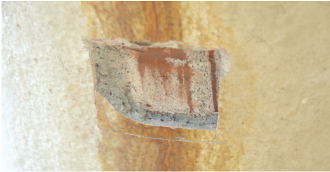
Image: PPG PITT-CHAR XP coating intact with excellent adhesion and corrosion protection after 13 years in service offshore
