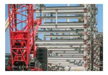
Both flexible and tough, PGG PITT-CHAR XP resists cracking and damage during slinging and handling, so that the fireproof coating remains in good condition when steel is transported and erected on site.
