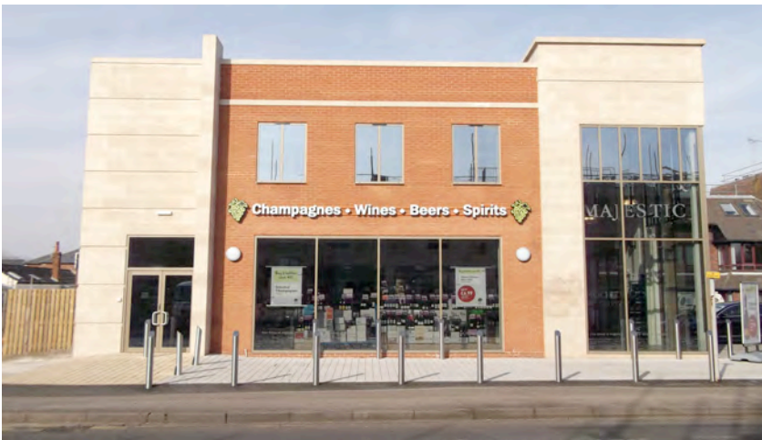
The contrast between the cast stone – which entirely replicates natural stone – and the red brick is striking.
