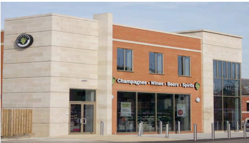
The rebated edges on some of the walling creates a very effective shadow-gap.
