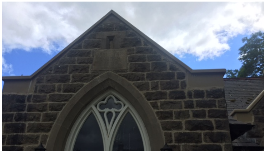
The original natural stone walling is complemented by the new cast stone
