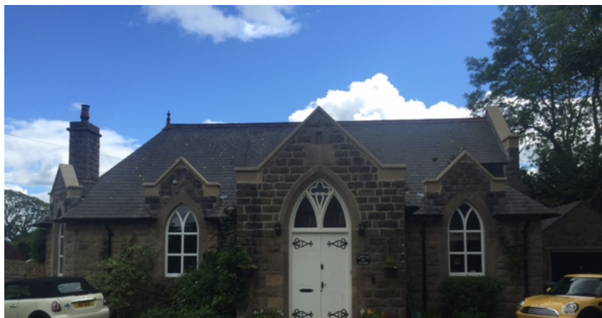
Coping and kneeler blocks were supplied to all the gable features
