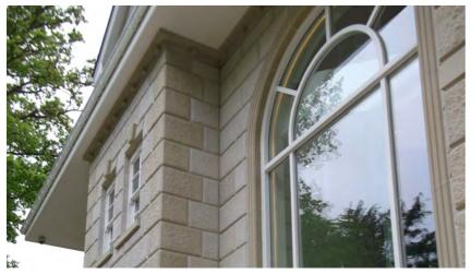
Close-up showing the excellent detailing of just some of the cast stone units.
