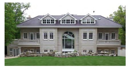
This substantial new residential property has cast stone as the main external building material.
