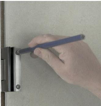
When the shower door is in place placed, mark the three screw holes in both wall hinges with a pencil. The marks must be precise and clearly visible when the shower door is removed
