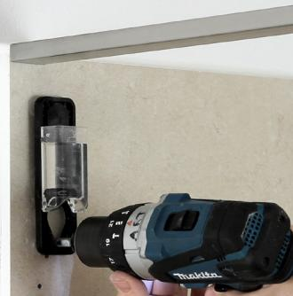
Remove the shower door and drill the marked points with a 6 mm tile bit.
