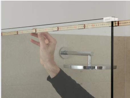
Measure the depth of the shower cubicle from the tiles on the wall to the unidrain® glass bracket.
