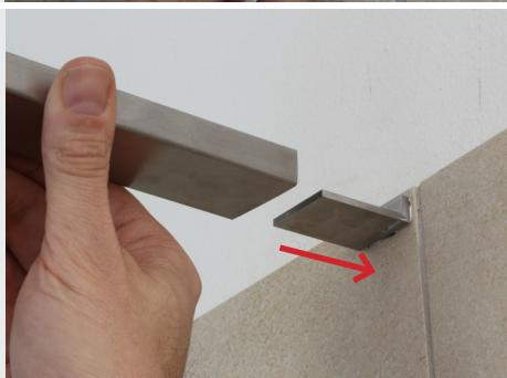
Slide the top rail carefully on top of the wall bracket.
