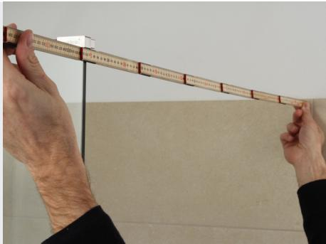
Measure the distance from the glass bracket to the tile wall on the opposite side.
