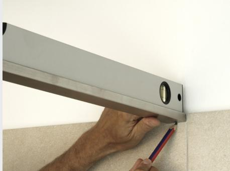
Hold the top rail horizontally using a spirit level and mark the tiles around the top rail.
