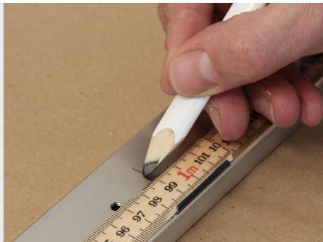
Mark the measurement on the top rail.
