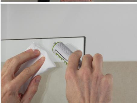
Lastly, any remaining silicone can be removed using silicone remover.
