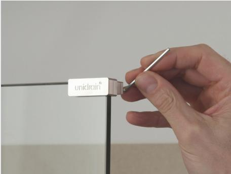
Place the glass bracket for the top rail on the corner of the shower screen and tighten it in place with the two set screws in the bracket.
