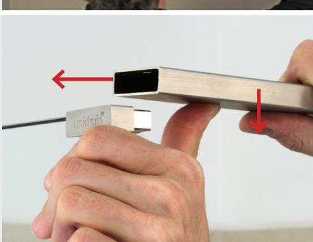
Place the cut top rail in the glass bracket by pulling the shower screen to the side so that the rail can slip into position.
