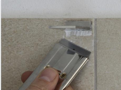
When the foam block is removed, there may be some excess glue residue that must be removed with a scraper or a utility knife.
