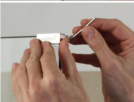
NOTE: Tighten the screws until there is resistance, and then a quarter turn more. The bracket is then attached in place.
