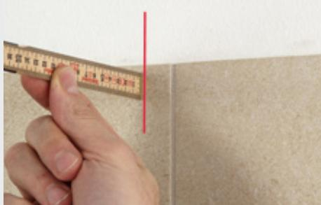
Use the exact place where the top rail will be installed when measuring.
