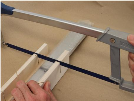
Cut the top rail with a hacksaw and preferably using a mitre box (**NOTE: Be careful not to scratch the steel**).
