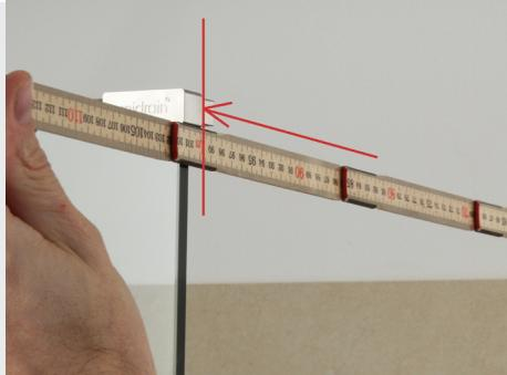
Only measure to the point where the top rail will rest in the glass bracket.
