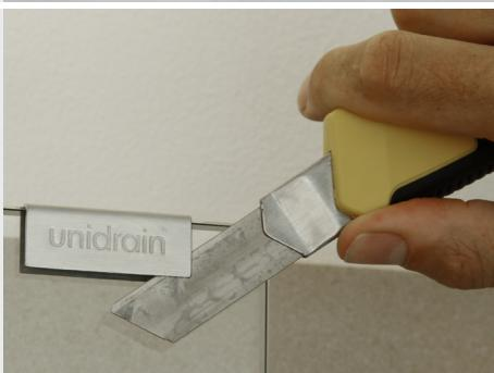
The unidrain® logo is glued on with silicone. Carefully cut the silicone loose using a utility knife (NOTE: Be careful not to scratch the glass).
