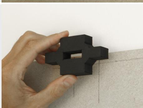
Remove the film on the foam block and fix the block to the tiles.
