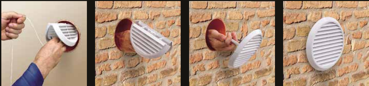
Fold the outer grille. Push through the wall tube. Open up the outer grille. Pull back on the string to secure to the outside wall.
