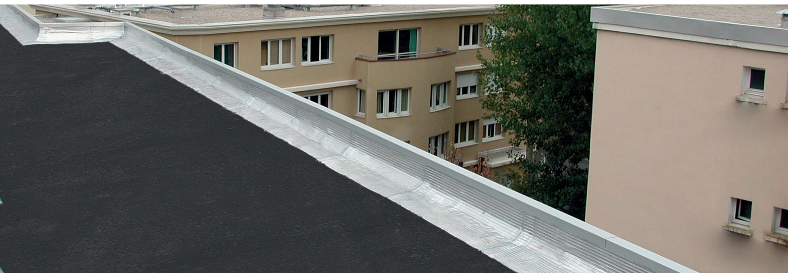
Example of an upstand parapet with reinforced protection (inside view)
