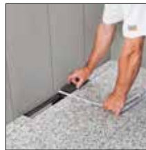
For 4. Measure covering for the covering support...
