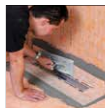
Fig. 4. Adhere Schlüter®-KERDI collar with Schlüter®-KERDI-COLL-L
