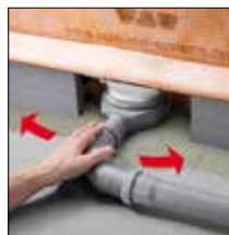
Fig. 5. Align the drain pipe
