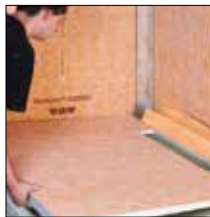
Fig 3. Slide the sloped tray under the edge of the channel body
