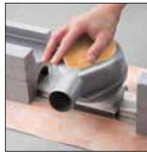
Fig. 3. Place drain body on adapter
