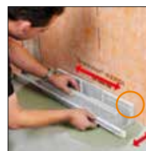
Fig. 1. Align the channel support
