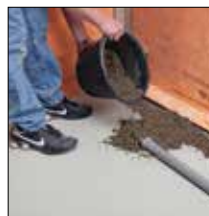
Fig. 6. Apply sloped screed
