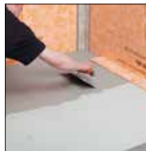
Fig 6. Apply thin-bed adhesive
