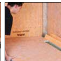
Fig. 3. Slide the sloped tray under the edge of the channel body
