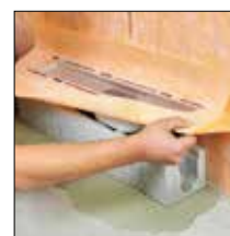
Fig. 2. Insert the channel body
