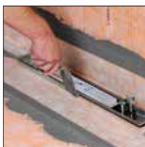
For 3. Fill frame/fully embed tiles
