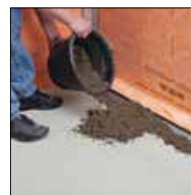
Fig. 3. Apply levelling screed
