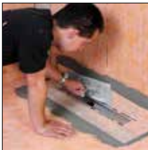
Fig 4. Adhere KERDI collar with KERDI-COLL-L
