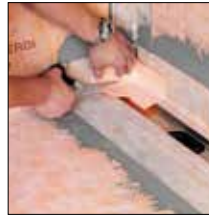
For 2. Adhere KERDI collar/ cut KERECK internal corner to size
