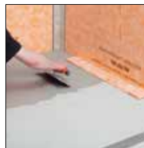
Fig. 7. Apply thin-bed adhesive
