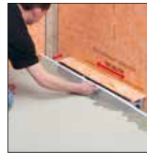
Fig. 4. Align the channel support
