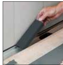
For 2. Insert spacers into the channel body
