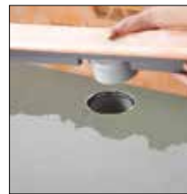
Fig 4. Attach channel body with channel support
