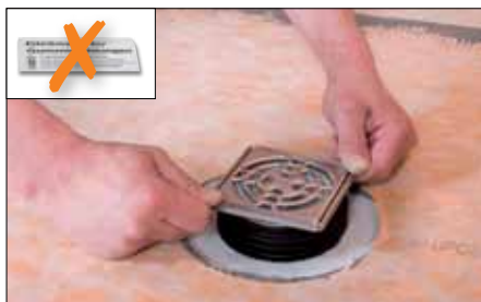
21 Slide the stainless steel grating assembly into the bonding flange.
