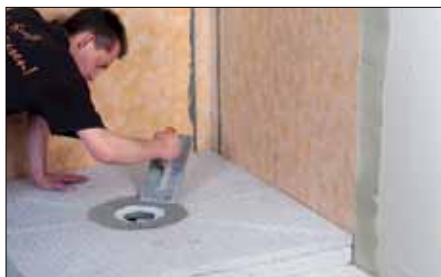
16 Apply Schlüter®-KERDI-COLL to the flange of the bonding flange.
