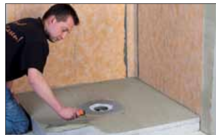
17 Apply thin bed adhesive to the remaining area with a 3 x 3 mm or 4 x 4 mm notched trowel.
