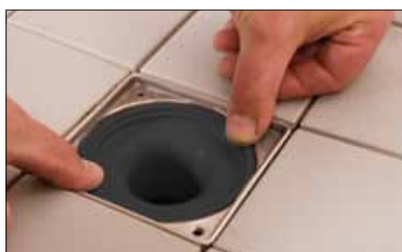
23 Prior to using the shower, remove the stainless steel grating and press on the odour trap to check its positioning (if necessary, apply some lubricant to the O ring).
