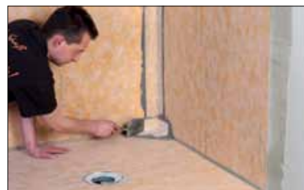
20 a Fully embed the prefabricated corner pieces in Schlüter®-KERDI-COLL.
