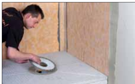
15 Push the bonding flange into the drain body and into the adhesive bed.
