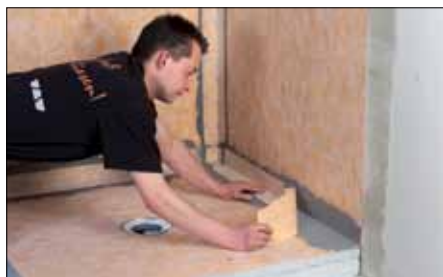
20 b Use Schlüter®-KERDI-COLL to tightly seal the wall connections with Schlüter®-KERDI-KEBA.
