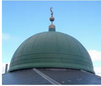
GRP structures can be manufactured to specific designs and sizes as shown in these examples.
