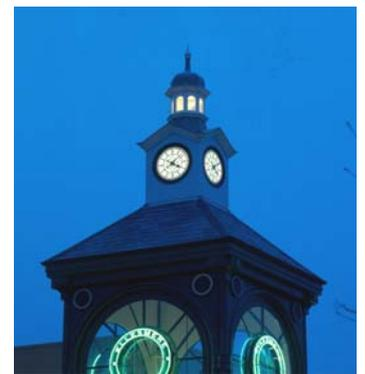
The clock tower below was copied from the original and now has pride of place back above a restaurant in Bournemouth. A unique feature of this 3m high cupola is that it actually rotates through 360°. Three sides have radio controlled lithium battery clock mechanisms. The fourth side has a window for a camera obscurer. This projects a view of the surrounding precinct onto a table below.
