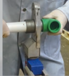
Heat up pipe and fitting
