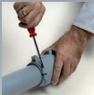
Insert pipe into fitting and tighten screws
