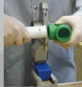
Bring the parts to be welded together
